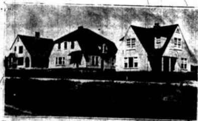
The three homes in course of construction—Left to right: Home of Overton Robnett, home in course of construction, for sale, and home of Marshall G. Clark.
