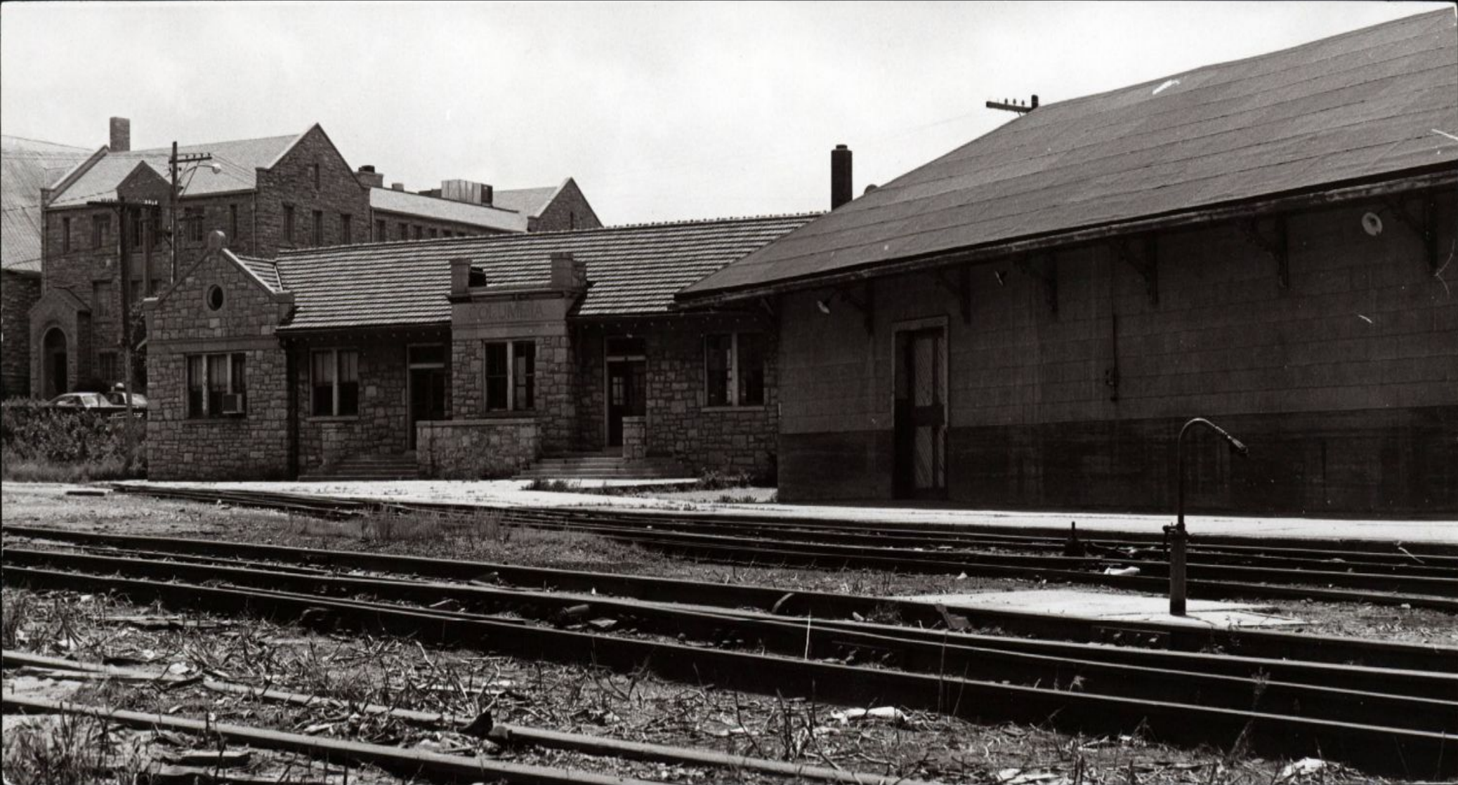
Wabash Station And Freight House 1970
